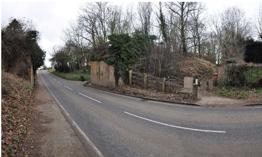
The crossing looking north east. The location of the original bridge can be seen.
