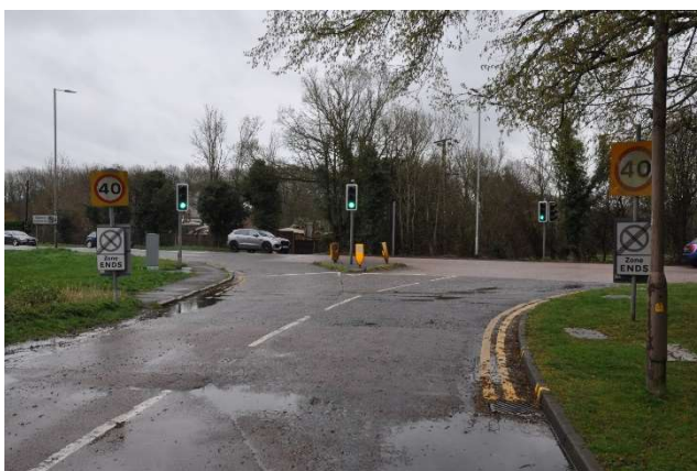
Dunmow Road / Thremhall Priory signals
