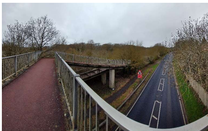
The footbridge at Hassels Lane (point 70)
