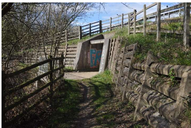
The mouth of the subway from the east
