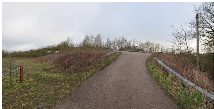
Bridge from Little Dunmow side
