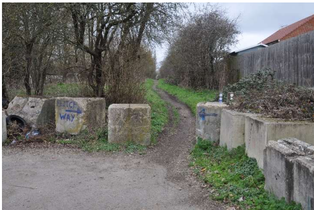
At traveller's site, Flich Green (point 88). Width not checked. Should be either, arranged to give a 1.5m gap, or, replaced by a line of bollards.
