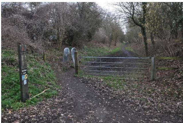
Buttleys Lane (point 59). The A-frame should be replaced by a 1.5m gap. To improve the alignment the vehicular access gate could be moved south (to the right of the picture).
