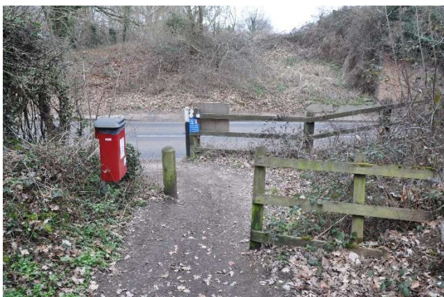
Station Road, Flich Green (point 89). The need for something like this chicane here is understandable due to the 40mph road with poor sightlines and downhill approach. But the chicane would filter out disabled scooters and the LTN 'design cycle'. Ideally the original bridge should be replaced and this access made pedestrian only with a hunting gate set back from the road.
