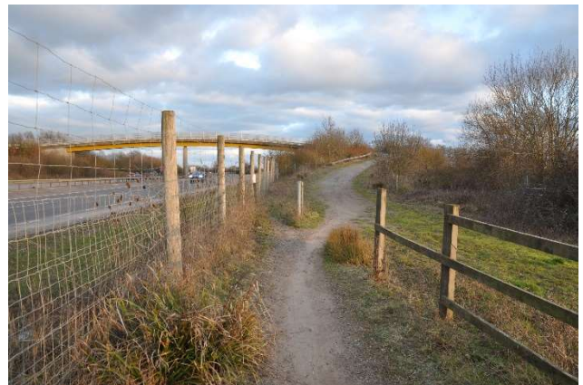
Looking east. A120 bridge (58) in distance
