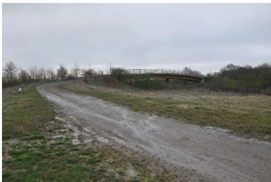
Bridge from Bumpstead Hill side
