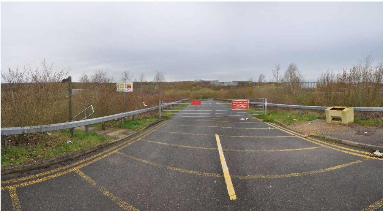
North end of footpath at A120. Steps down to left, gated road to Balancing Ponds, ahead, and footway over A120 bridge to right (point 21).
