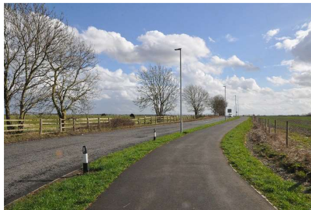
Clay Lane, Warrington – fence line set back to create space for cycletrack
